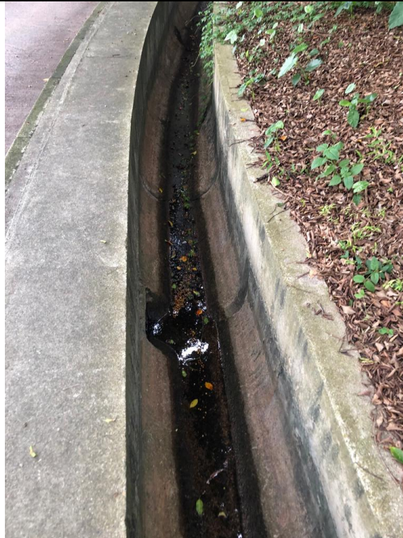
View 2 Existing 600UC within 300x 300 underground drain
