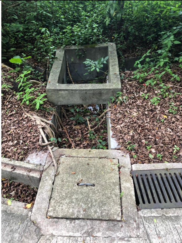
View 1 Existing 225UC and Catchpit
